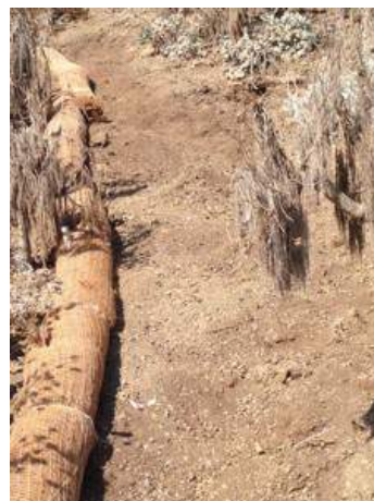
Wattle in Place
